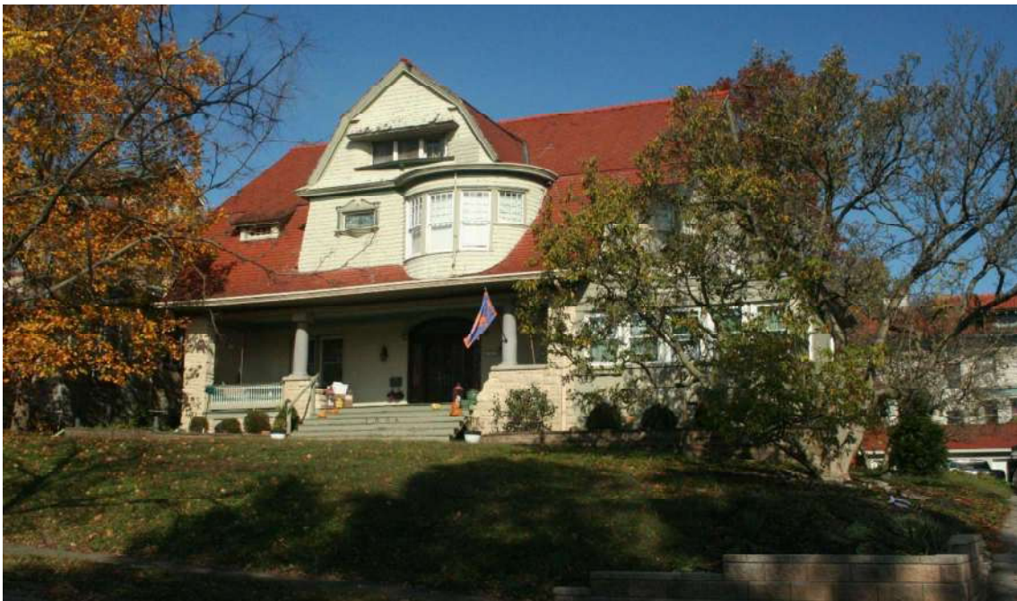
Photo 17. 1006 Lenox Place (1900), Shingle style.
