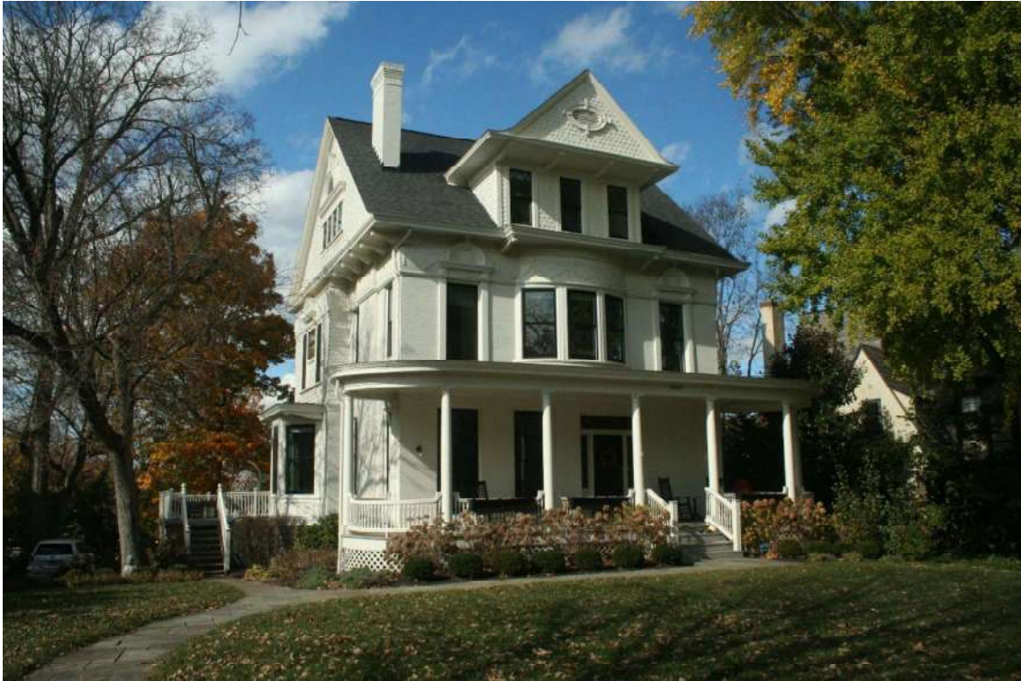
Photo 16. 3987 Rose Hill Avenue (1894), Stephen R. Burton House), Queen Anne.
