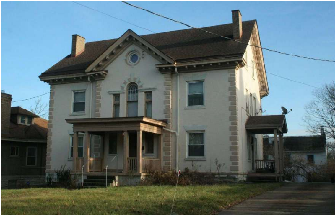
Photo 26. 3818 Dakota Avenue (1920), Georgian Revival.
